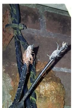
He then reported that the external grade shielded Ethernet cable for the 5GHz Link had also been badly chewed. As we were loosing light, several pictures were taken of the area so we could closely inspect the damage.
