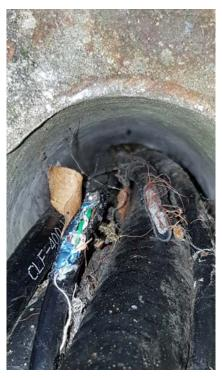
to a pre-made standard drop cable. The new cable connection was tested and bingo, our link was re-established. Outside lashings of Denso tape was applied to water proof the work around and the cable portal temporarily blocked to stop the return of our diner.
